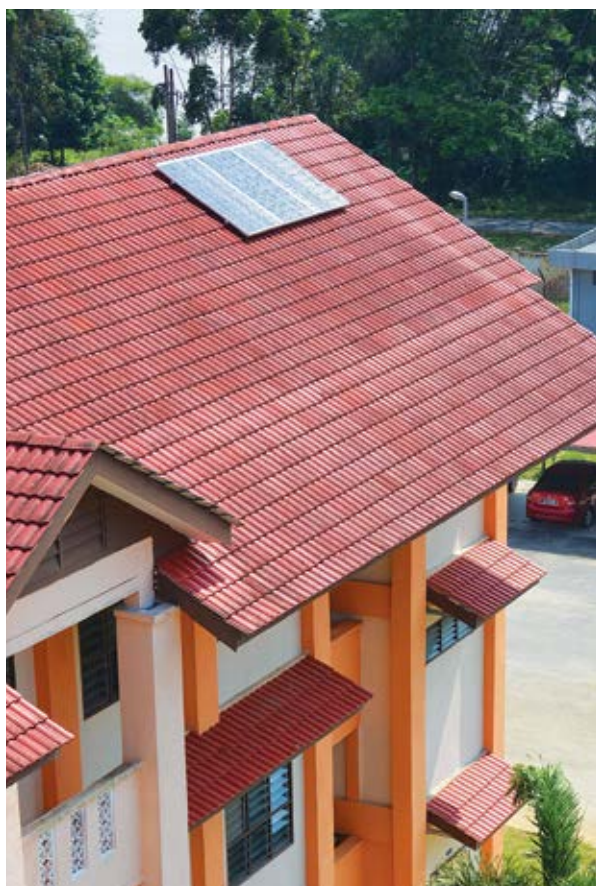
Solar panels were installed in SK Tebing Tinggi, an evacuation centre, to ensure a safe haven for evacuees in the event of a flood
